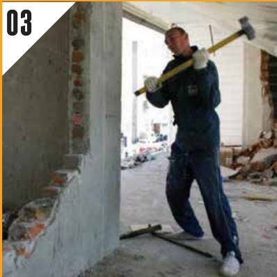
結構還原 Rebuild Building Structure
