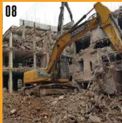
工業大廈拆卸 Demolish Industrial Building
