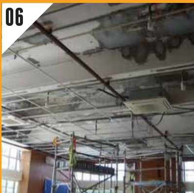
寫字樓清拆 Office Demolition
